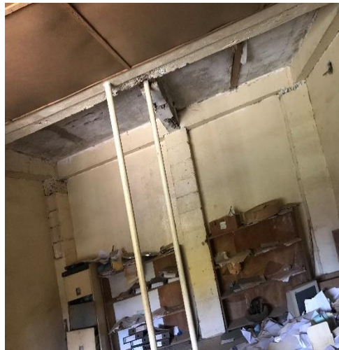
Photo 16: showing slab, column that have cracks
