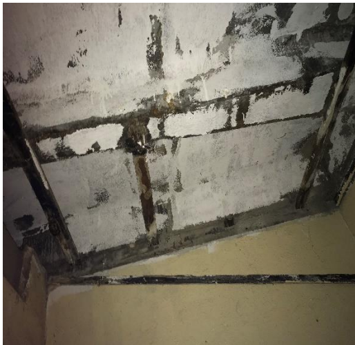
Photo 15: showing rusted rebar from slab
