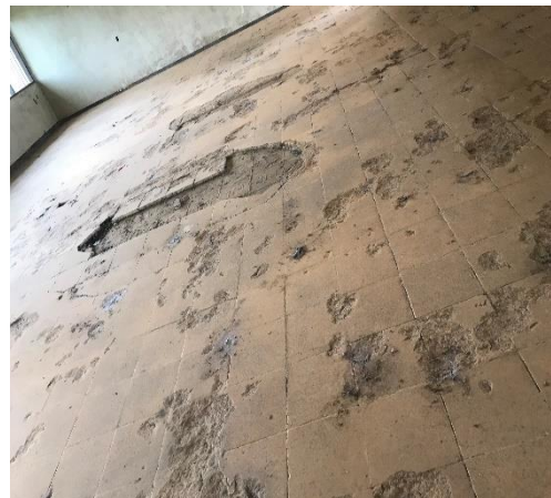
Photo 08: showing damaged terrazzo floor tile
