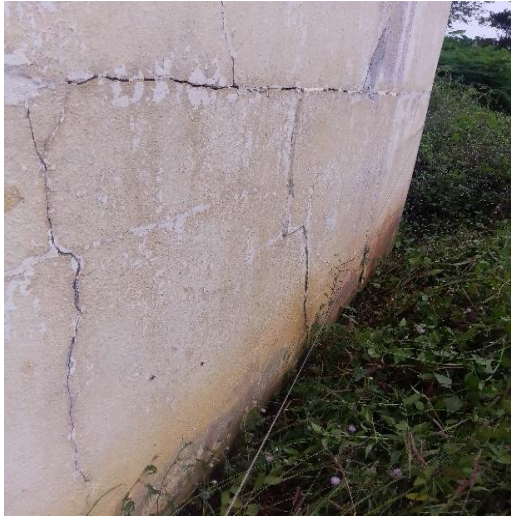
Photo 33: showing cracks on the boys dormitory
