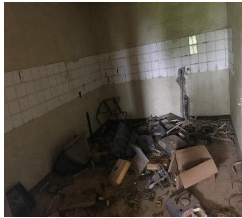
Photo 06: showing room with broken wall tile
