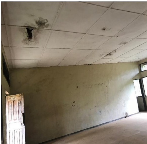
Photo 03: showing damage ceiling & sign of leakage
