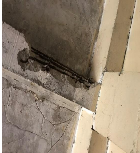
Photo 18: showing cracks on slab and rebar
