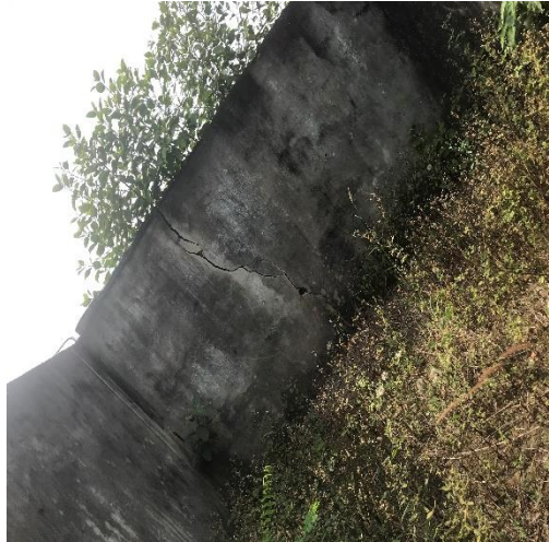
Photo 38: showing crack on wall of student center
