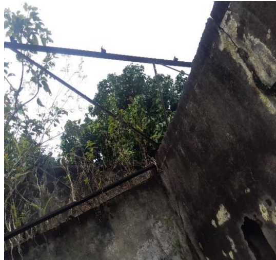
Photo 30: showing rusted steel trusses
