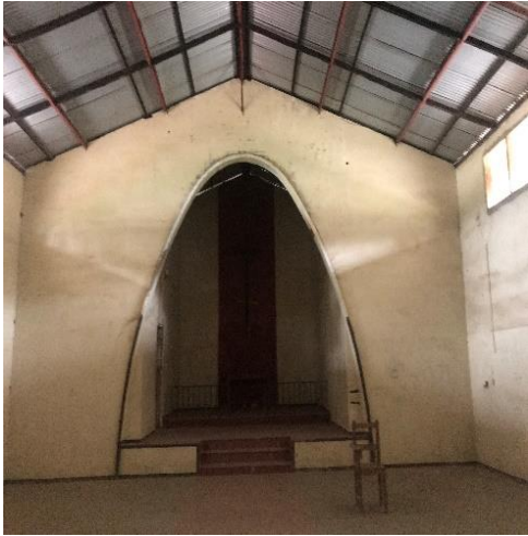
Photo 09: showing walls, roof and no ceiling in chapel
